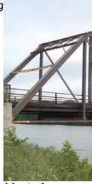
Built in 1908, the former two-span Pennsylvania through-truss bridge was the oldest of its kind in Wisconsin.
